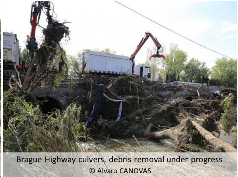
Brague Highway culvers, debris removal under progress © Alvaro CANOVAS
