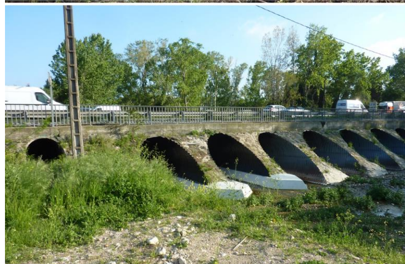
Brague Highway culvers in normal state Jul. 15, 2015 © G. PITON IRSTEA
