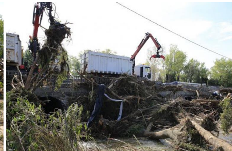
Brague Highway culvers, debris removal under progress © Alvaro CANOVAS
