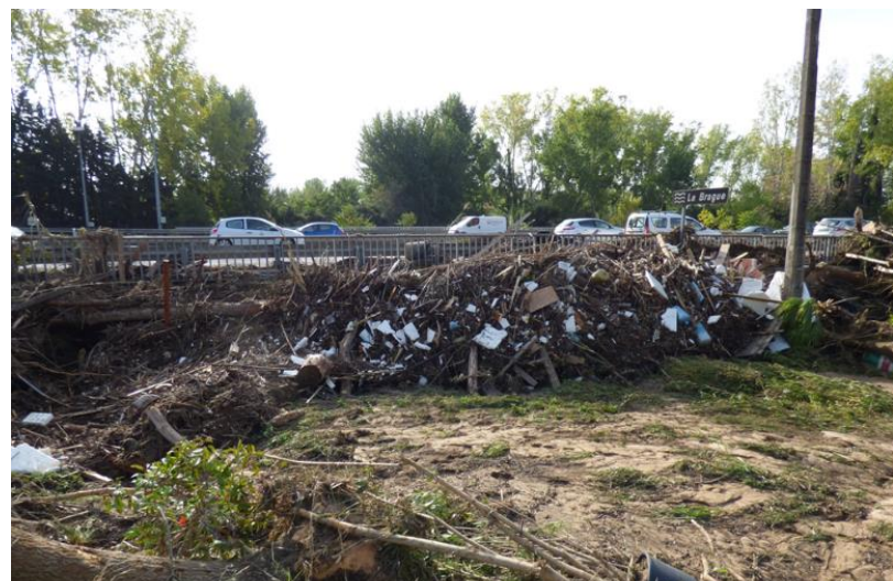
Brague Highway culvers submerged by wood and trashes © B. CARDELLI DDT06
